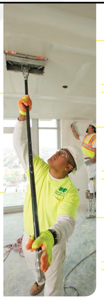
Finishing boxes consistently dispense the appropriate amount of joint compound and feather both edges in a single pass.
